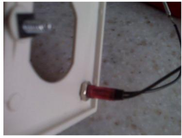
new 2x4 inch electrical box. Then I added a switched plug combo to the new box. To know when it was switched on or off, I added a red led to light up when the switch was in the on position.
